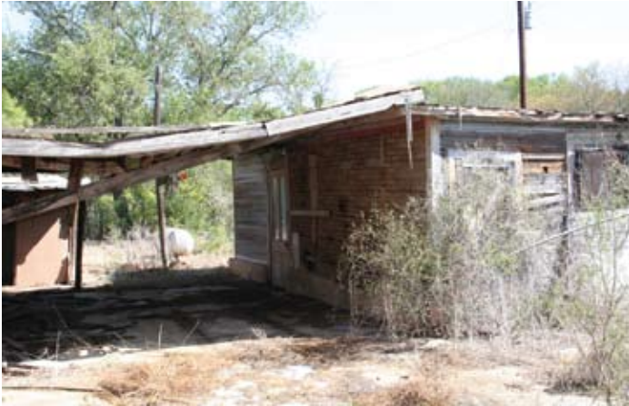
Fig 1. Hive entrance facing carport.
